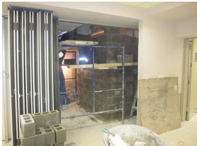
Progress continues as indicated above. The Foundation and the Concrete Roof have been completed. Interior work has begun with the Elevator Shaft construction and the opening of the existing Fellowship Hall Wall into the new space under the parking lot. See more Photos on the Church's website, [www.stnicholasalbanian.org](http://www.stnicholasalbanian.org). On the homepage, click the "Construction Progress" box at the lower right corner.
